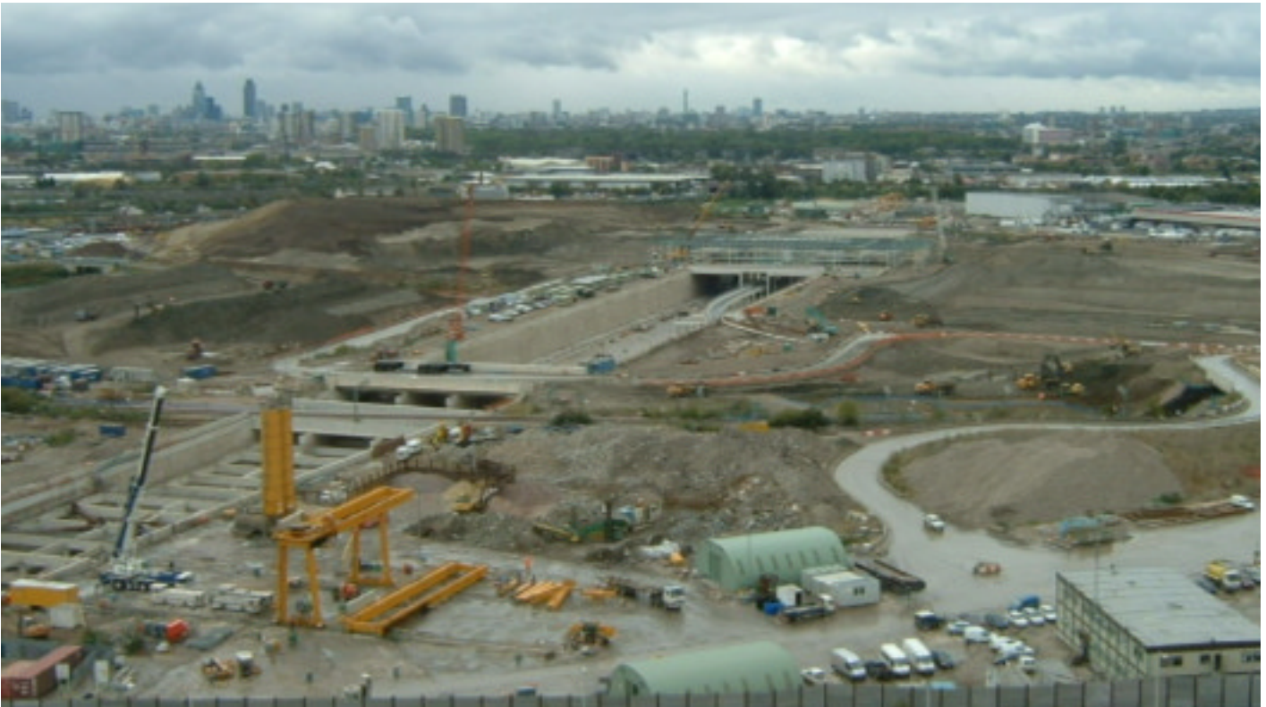
The Stratford City site covers 73 hectares and has Stratford International station at its heart.
